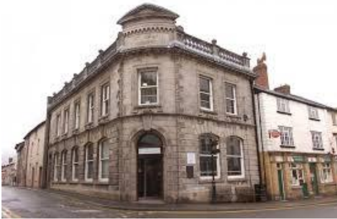
Head office of the Old Radnor Trading Company
