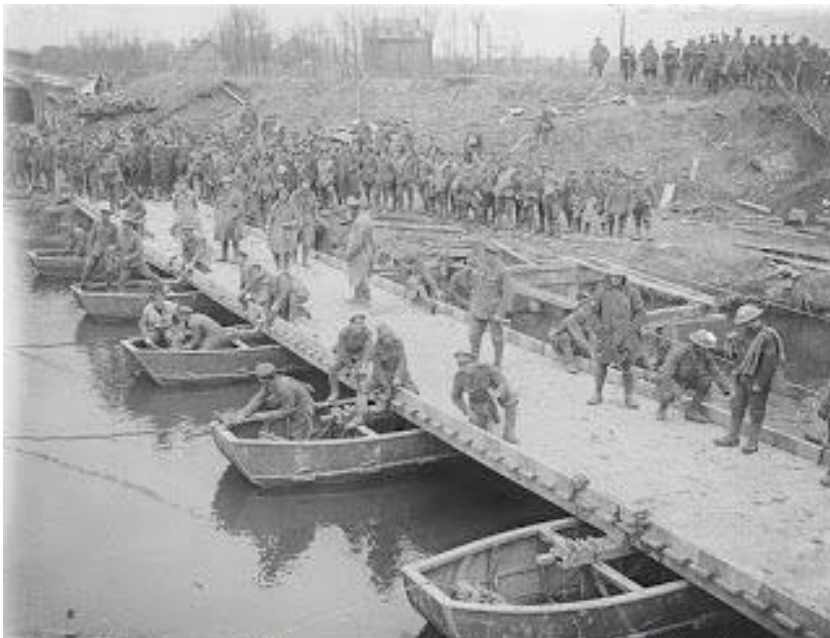
Royal Engineers build a pontoon bridge across a Belgian river
